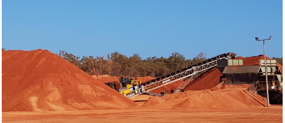
Figure 4. Barge Loadout infrastructure: Top - screening and feeder, Bottom - barge loader
