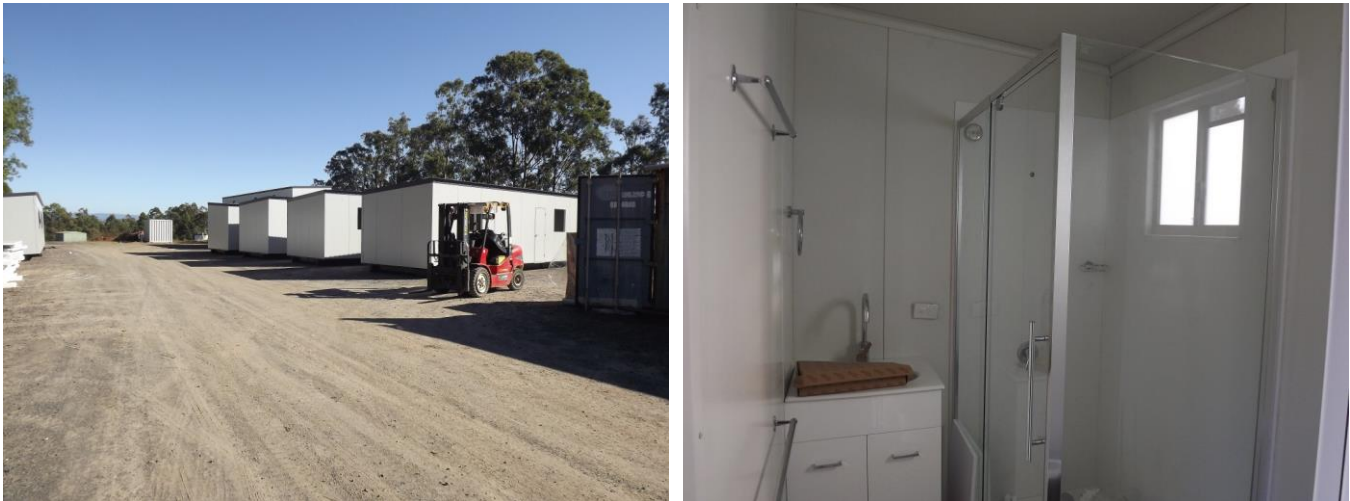
Figure 4: Bauxite Hills Mine accommodation village construction in Gatton, Qld
