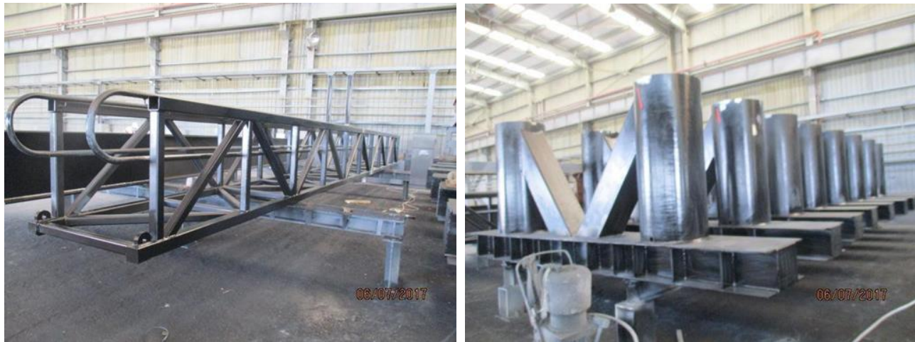
Figure 3: Fabricated steel on factory floor in China
